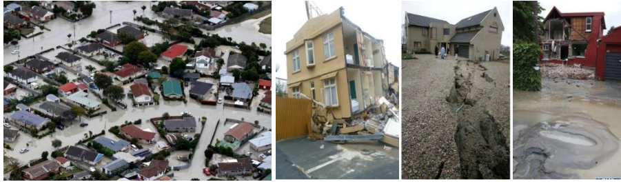
Fig. 2. The liquefaction damage in 2011 New Zealand earthquake
