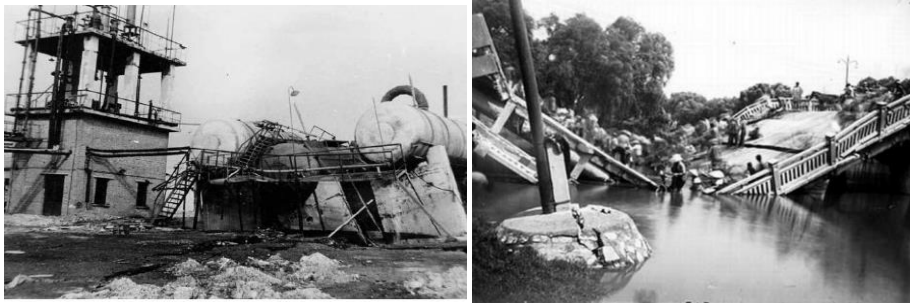
Fig. 1. The liquefaction damage in 1976 Tangshan earthquake
