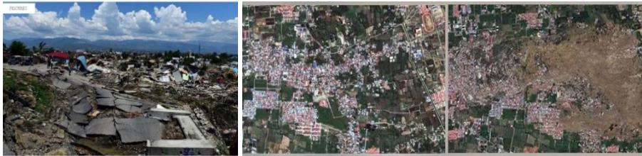
Fig. 3. The liquefaction damage in 2018 Indonesian earthquake
